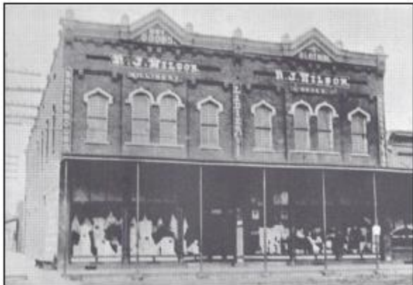
W. J. Wilson Store - 301 W. Main; built 1885
