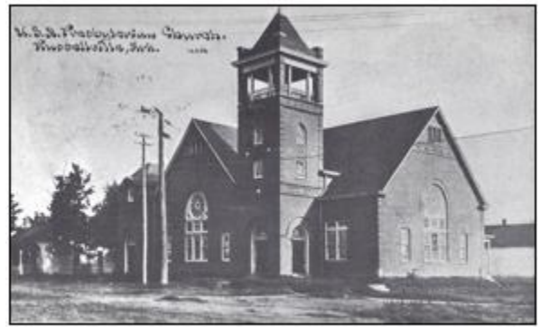
Presbyterian Church 1908 Building
