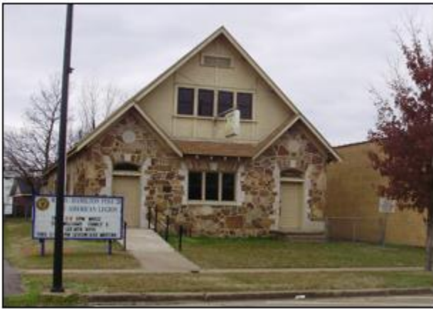
American Legion Building Fieldstone
