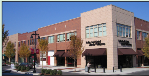
New buildings in Downtown Russellville should not exceed three stories. Mixed use and commercial buildings should be built up to the sidewalk.
