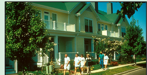
This building represents an attached housing type. The projections and recesses are effective in breaking up the facade mass.
