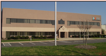
This facade's uninterrupted plane fails to achieve a human-scaled massing. It also has a horizontal orientation rather than a more appropriate series of vertical bays.
