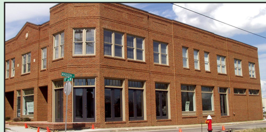
Flat roofs should be screened with a parapet facade on the building's frontage. The parapet should also screen rooftop equipment.
