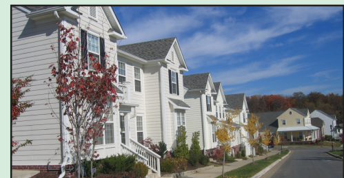
Varied roof lines are one tool for breaking up the massing of large structures. These roof forms are compatible with downtown.
