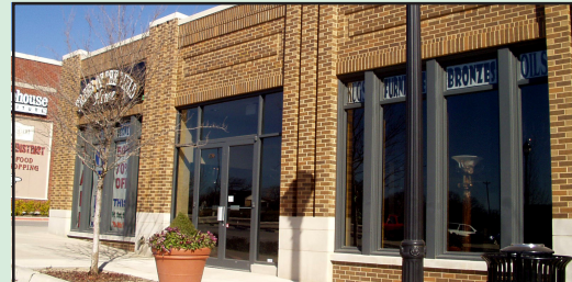
Pilasters (attached pillars), storefront windows, and cornice line variations on this new building break up the facade into vertically oriented bays.
